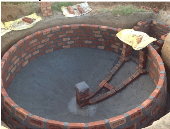
Our Biogas plant is almost ready after construction
