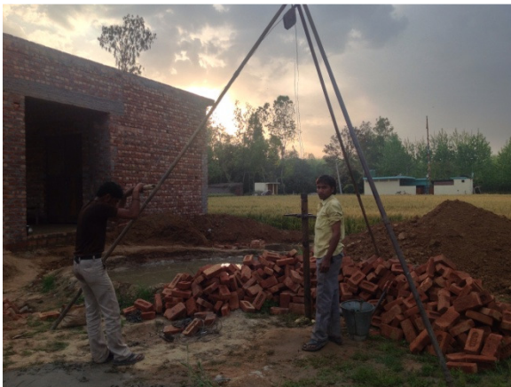
Our bore well of hand pump under drilling
